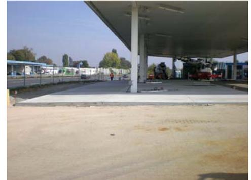
Examples of preventative measures taken by the industry to minimise risk of soil contamination: a bund and floor in a tank area (left) and a fluid-tight pavement being installed in a petrol station during construction (right). Investment in such measures is preferable to clean-up costs.
