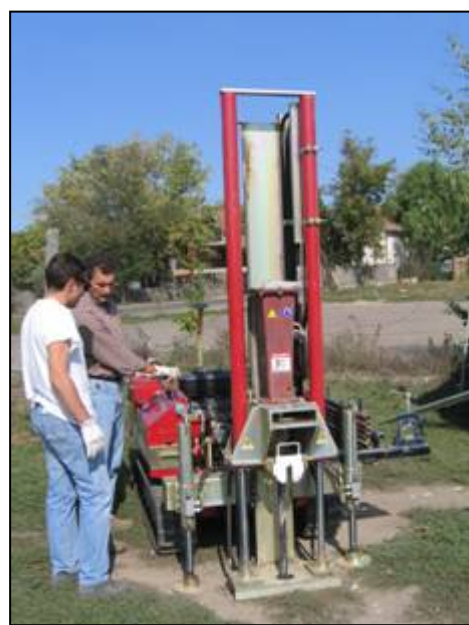
Direct Push drilling and in situ sampling of ground water on PCE with Geoprobe®.
